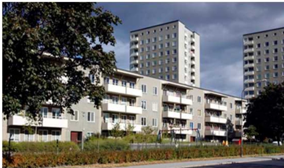
Photo: Refurbishment, Valla Torg, Stockholm
